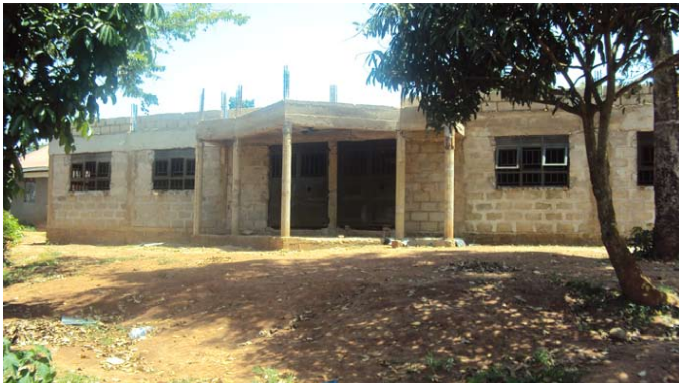
A longitudinal view of the building under construction at Masooli center
